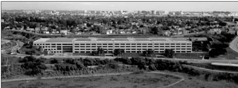
University Hall houses faculty offices, classrooms and many other facilities.
